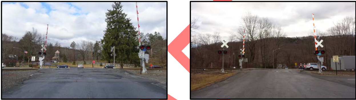
Figure 2 - Westbound and Eastbound View of Crossing
